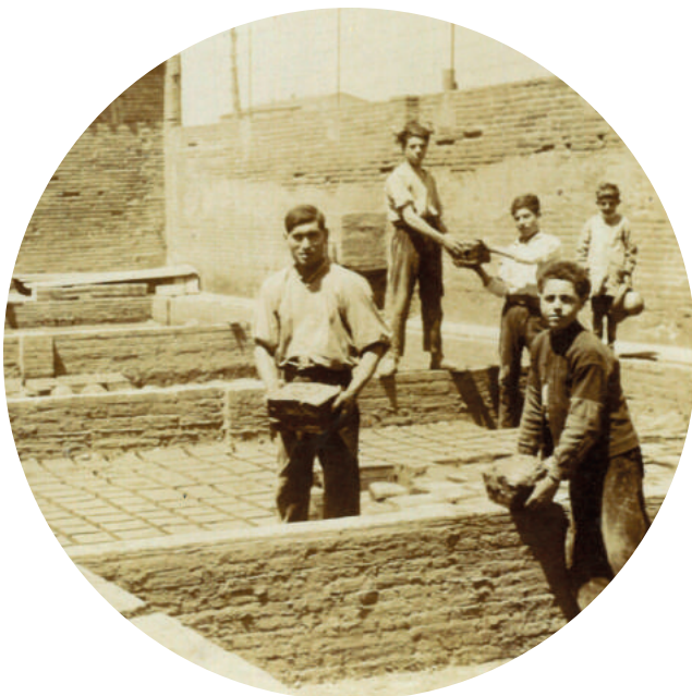
Preparation of clay in settling ponds in L'Hospitalet factory, early 20th century
